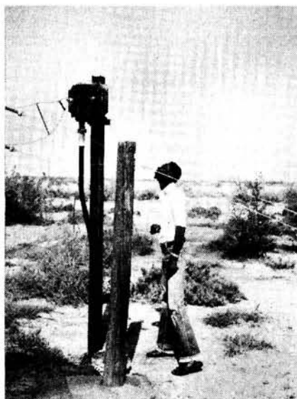
A communications technician in Mauritania (5T5-land) examines a 1kW balun unit that is connected between the 50Ω coaxial cable (seen coming out of the ground) and the feed-line on the log-periodic antenna
